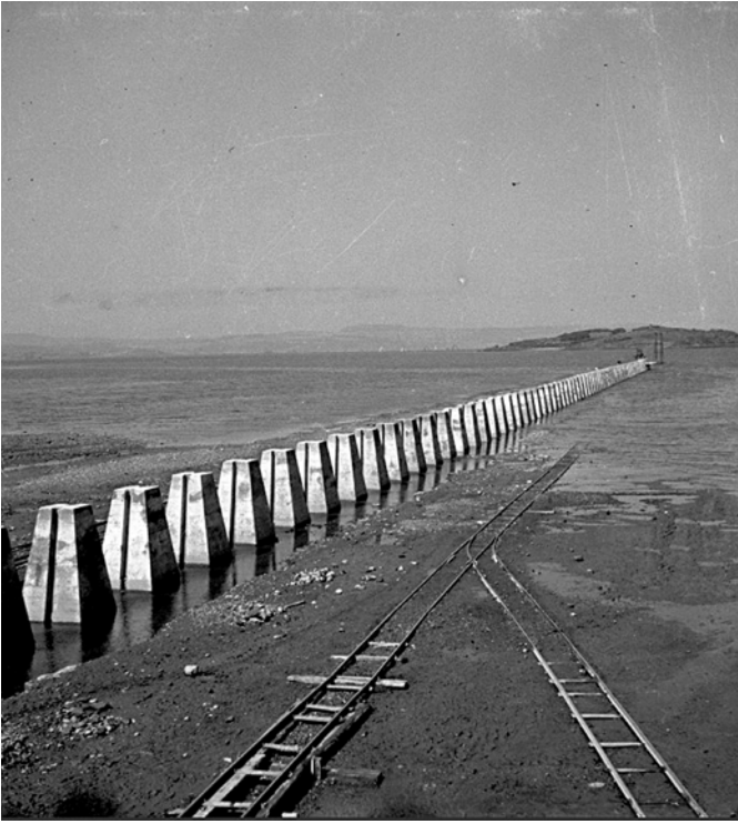
Views of the anti-ship ping shipping barrier running from Cramond to Cramond Island, showing construction work in various phases, 1940. Copyright Royal Commission on the Ancient and Historical Monuments of Scotland/Crown Copyright, OER
