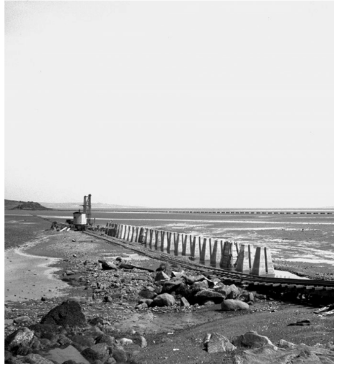
Views of the anti-ship ping shipping barrier running from Cramond to Cramond Island, showing construction work in various phases, 1940. Copyright Royal Commission on the Ancient and Historical Monuments of Scotland/Crown Copyright, OER
